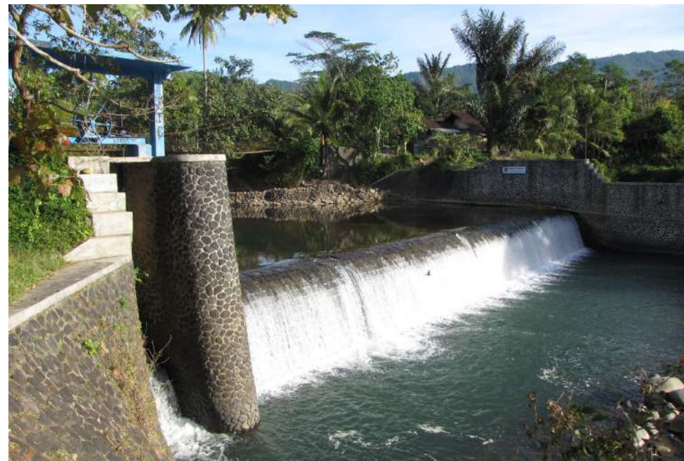
Tirta Gemah hydropower in Indonesia. Photo: Nefco
