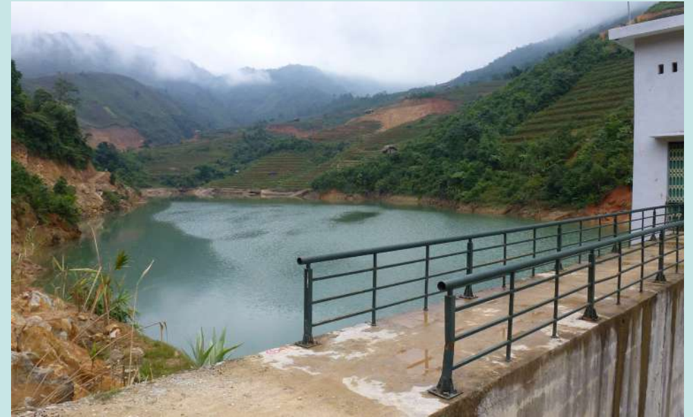
The water dam in Nam Khanh, Vietnam. The project generated 132,500 CERs. Photo: Nefco
